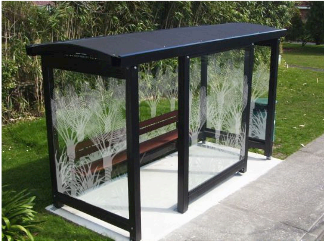
Figure 3: Standard North Shore City Bus Shelter with Planned Glazing Improvements
