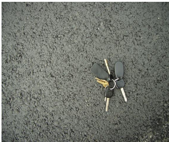
Photo 9: The surface of the RAP appeared dense and coherent.
