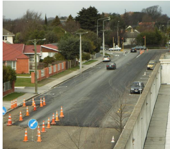
Photo 8: First 150m of the road paved with RAP, 8 July 2005.
