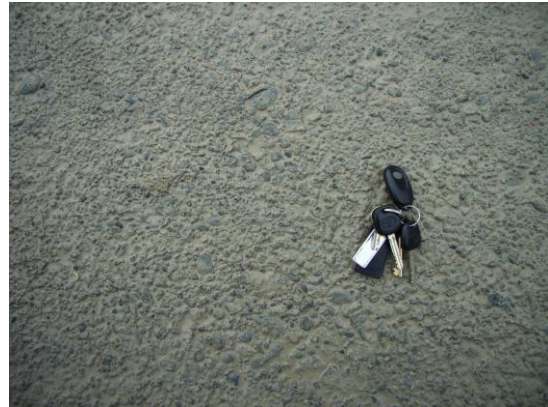
Photo 6: The surface of the AP40 basecourse ready for the 100% RAP topcourse.
