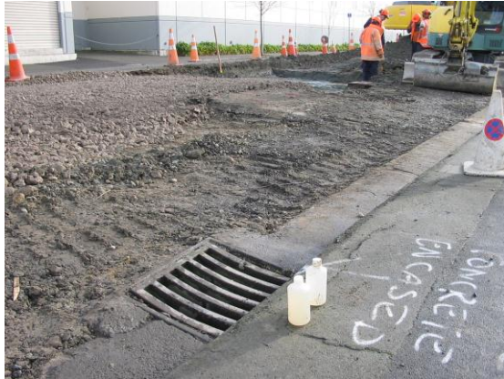
Photo 6: The surface of the AP40 basecourse ready for the 100% RAP topcourse.
