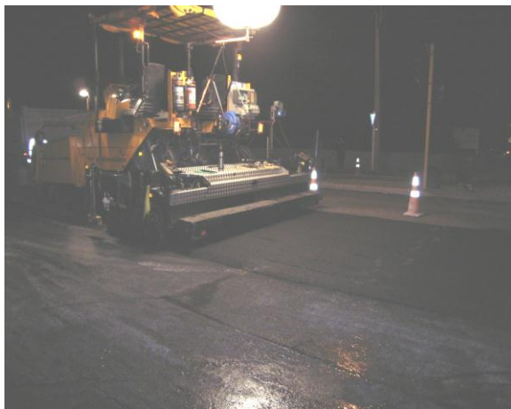
Photo 7: Night paving of the RAP mix, 7 July 2005.
