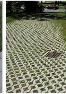
Permeable paving
