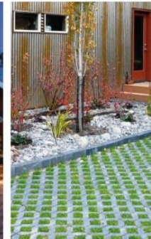
Permeable paving
