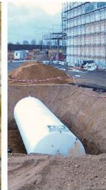
Subsurface rain tank
