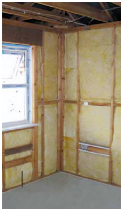
Fig 2. Light timber framed construction with Batt insulation
