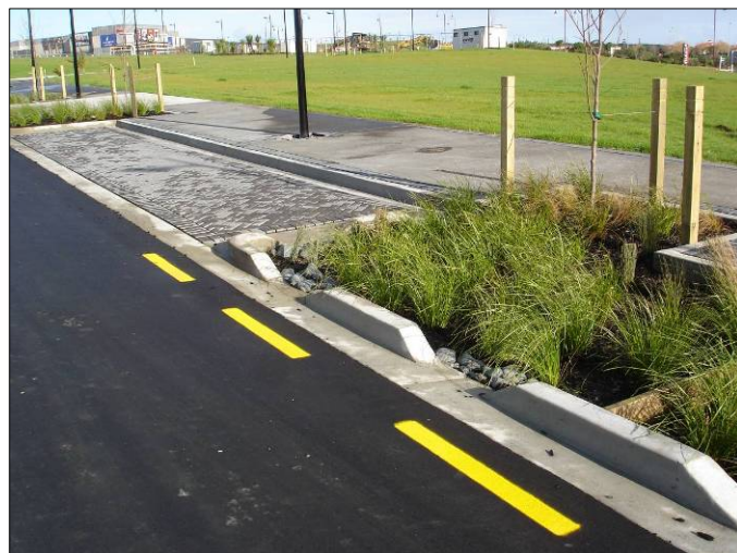
Figure 8: recently completed local street in Albany centre with permeable paving and a rain garden (bio-retention)
