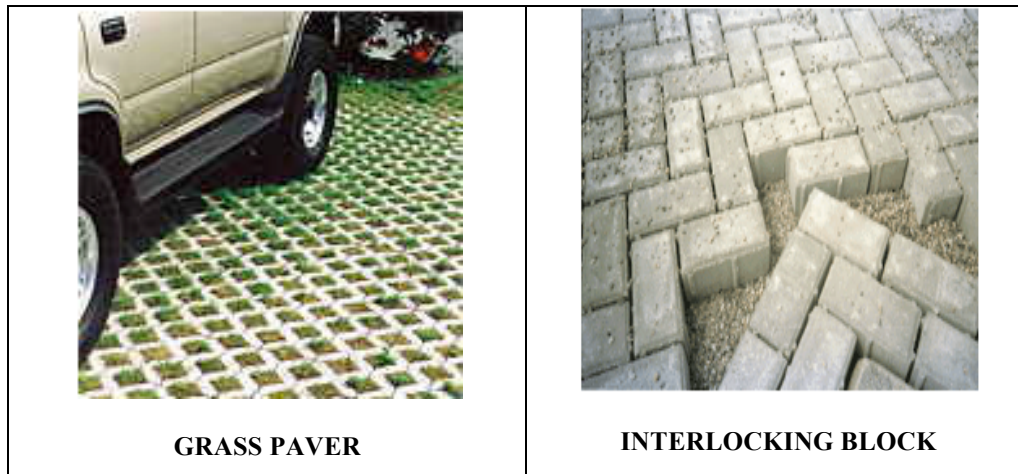
FIGURE 5: PERMEABLE PAVEMENT SYSTEMS
