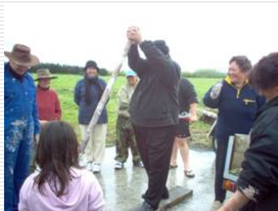
Cinva ram brick fabrication on-site in Te Toke NZ - photos courtesy of Bryan Innes
