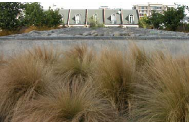
Environment Canterbury green roof (Landcare Research, 2008)
