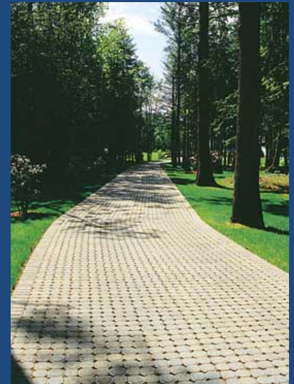
Permeable pavement footpath www.weneedsolutions.com
