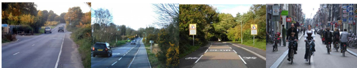
Figure 7 – Advisory cycle lanes in conjunction with removal of centre line (before and after in Felixstowe, England; The Netherlands – yes, cars can use this road)
