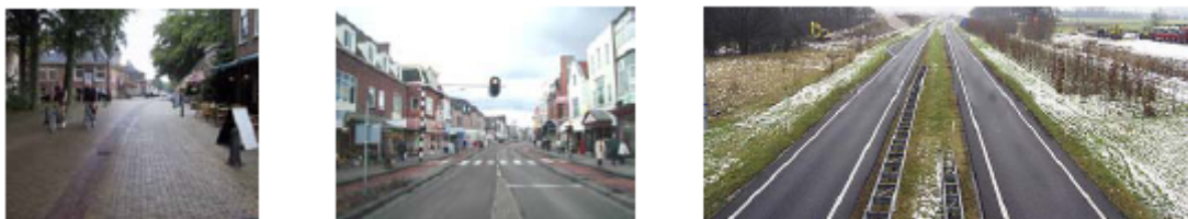
Figure 5 – Self-explaining roads (access road, distributor-collector road, through road)
