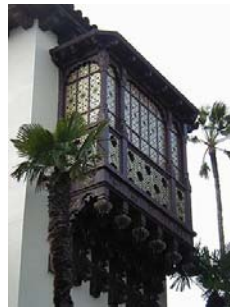
Fig. 22: Mashrabiya screen over a window in Coptic Cairo, side view (Golany, 1980)
