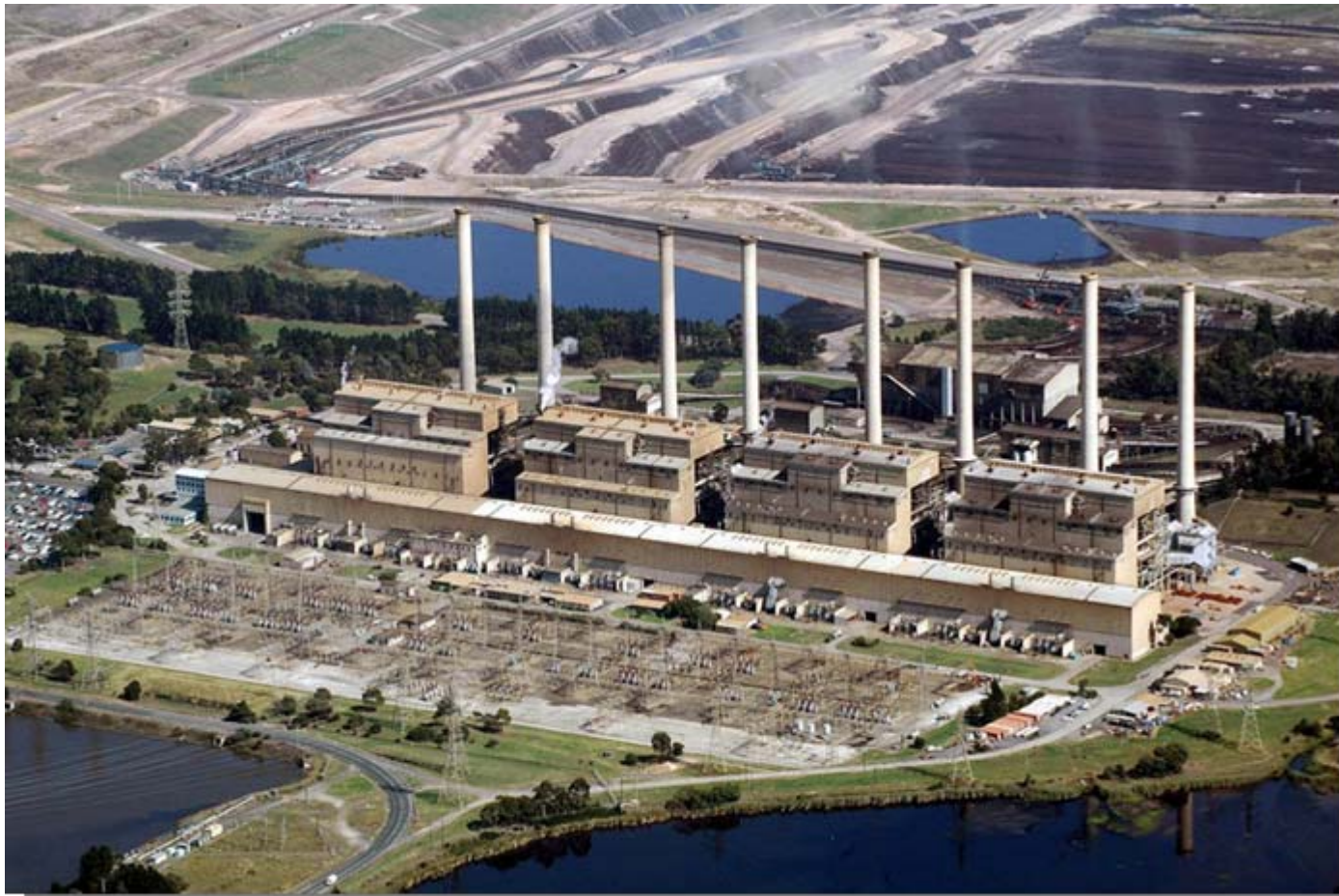
Hazelwood Power Station, Victoria (ABC NEWS, 2009)
